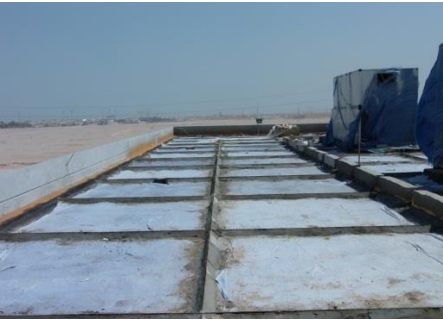
Water test & screed protection works 20 to 25 N opc300+Fibber
