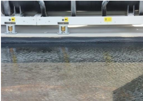
Applying SUPER WATERPROOFING RBE and GTEX 100 to 120 gsm Layer
