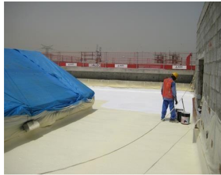
Applying SUPER WATERPROOFING RBE and GTEX 100 to 120 gsm Layer
