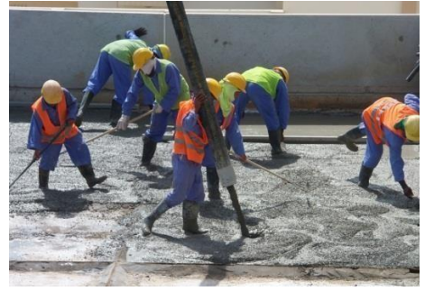
Water test & screed protection works 20 to 25 N opc300+Fibber
