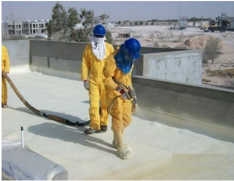
Applying SUPER WATERPROOFING RBE and GTEX 100 to 120 gsm Layer
