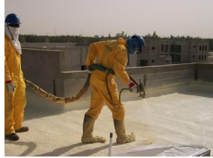
Prime proof / BCI/Bayer PU40 spray applied over the concrete slab
