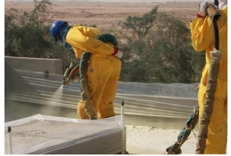
Prime proof / BCI/Bayer PU40 spray applied over the concrete slab
