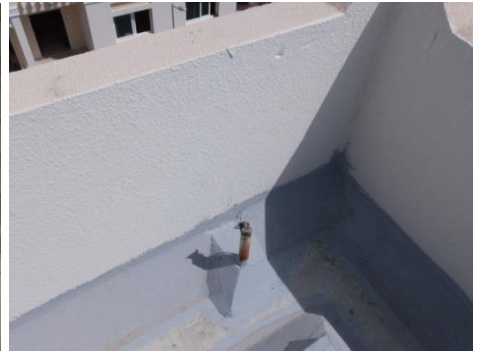
Applying SUPER WATERPROOFING RBE and GTEX 100 to 120 gsm Layer
